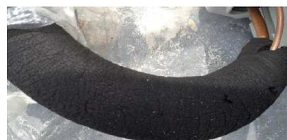
Prolonged exposure to the sun and environment causes cracks
