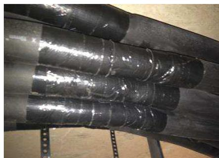
PVC tape wrapped around joints without glue
