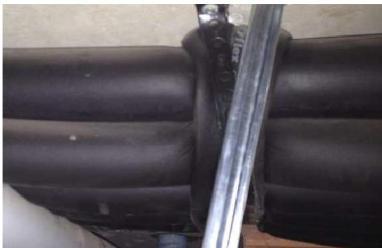
Example of pipe support reducing thickness and crowded pipes thickness
